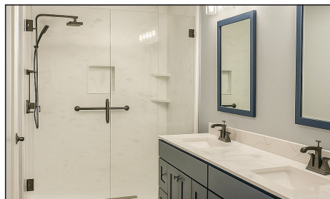
FULL BATHROOM REMODELS
